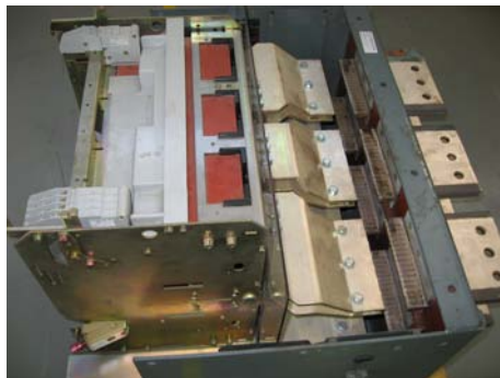
New w/drawable ACB installed into UNELEC C9 3150A ACB
