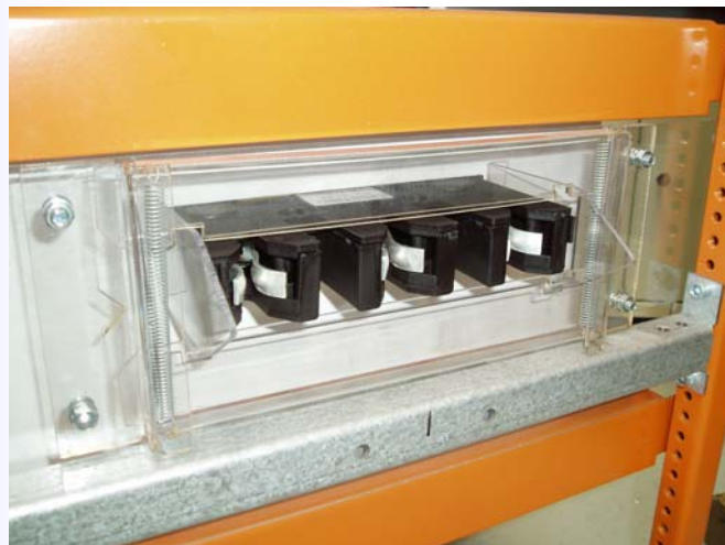
Busplug/tray partly inserted
